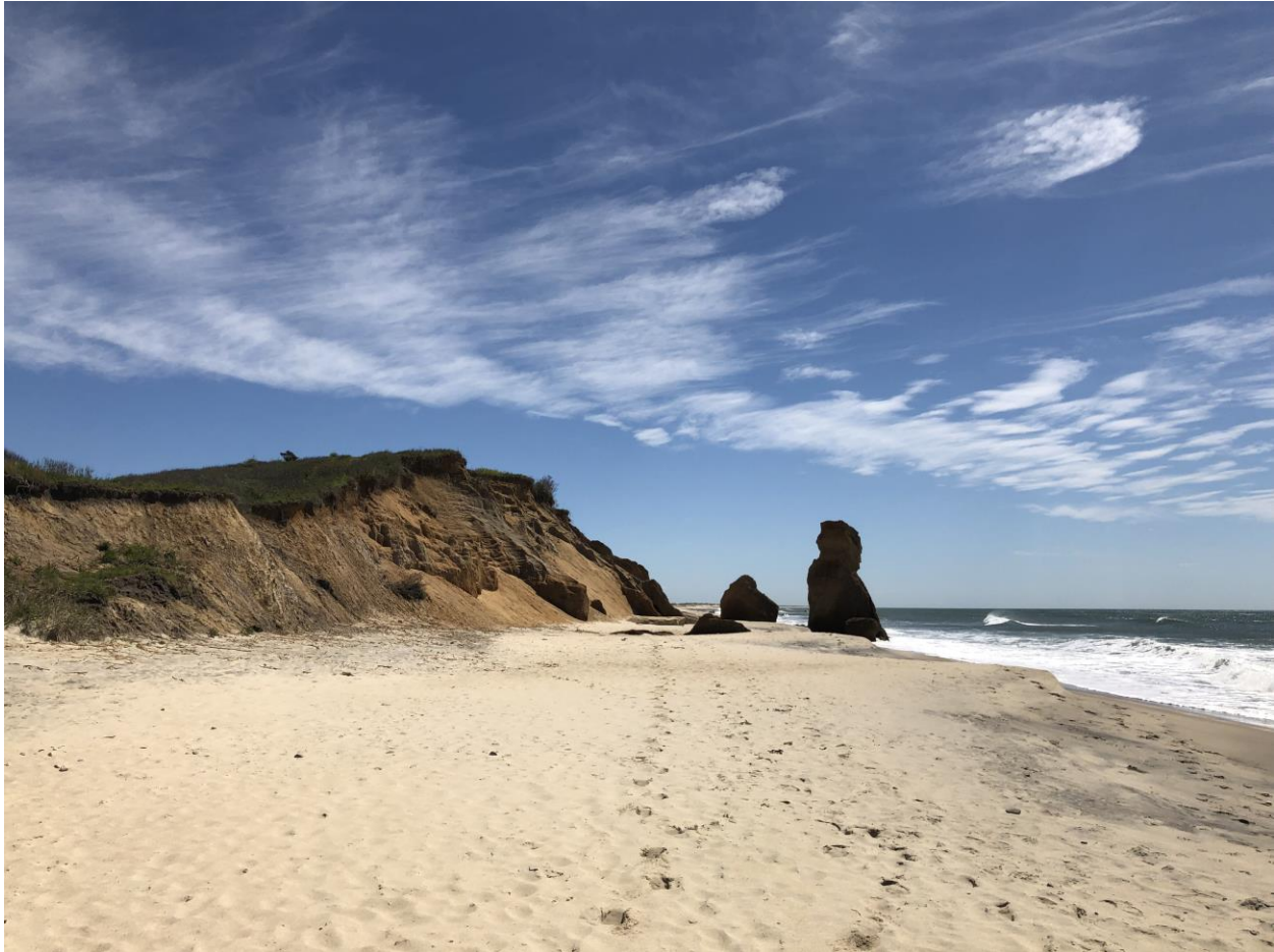
Figure 5. An example of a sandy beach backed by a tall coastal bluff in FEMA Region 1. Many bluffs in this Region have historically eroded.
