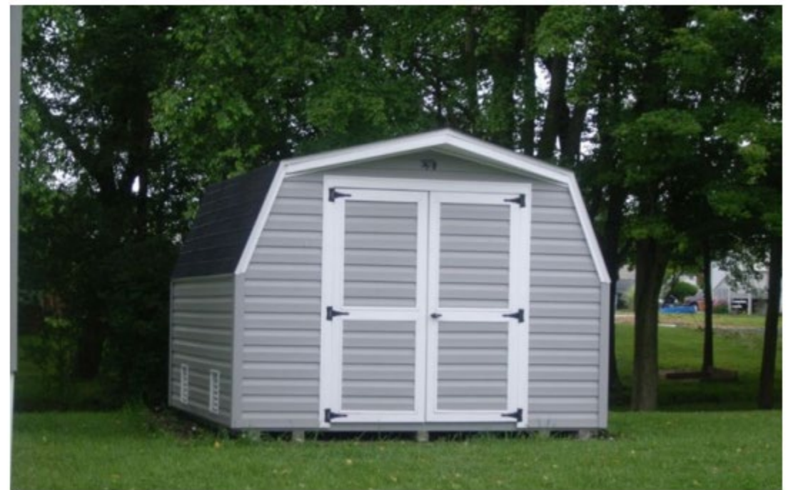
Figure 16: Storage Shed, with Flood Openings (Source: Kevin Wagner, Maryland Department of the Environment)
