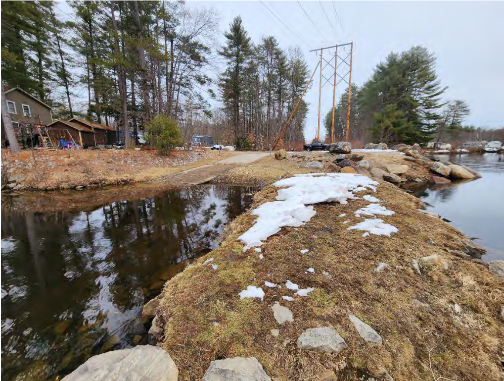
Figure 8. Boat Ramp upstream of Rolfe Canal Dam
