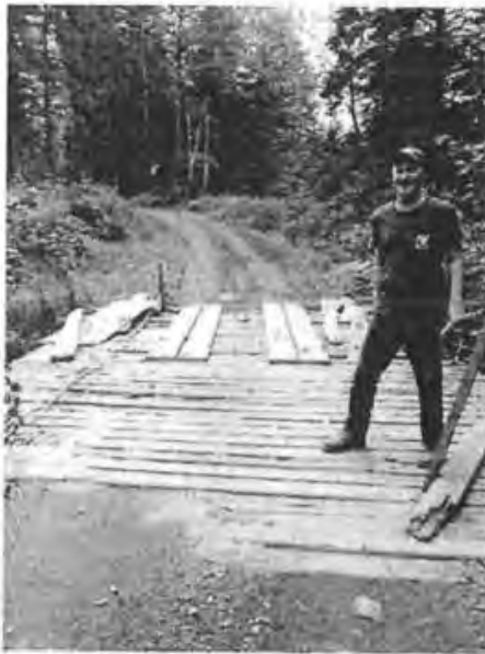
Figure 1 and 2- Shows the broken boards on the bridges that need to be replaced.
