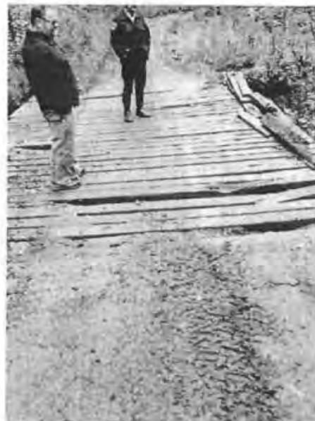
Figure 1 and 2- Shows the broken boards on the bridges that need to be replaced.
