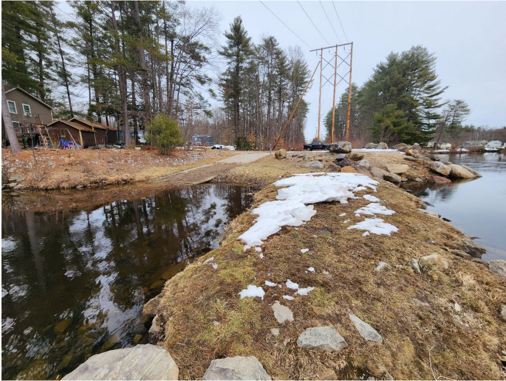
Figure 8. Boat Ramp upstream of Rolfe Canal Dam
