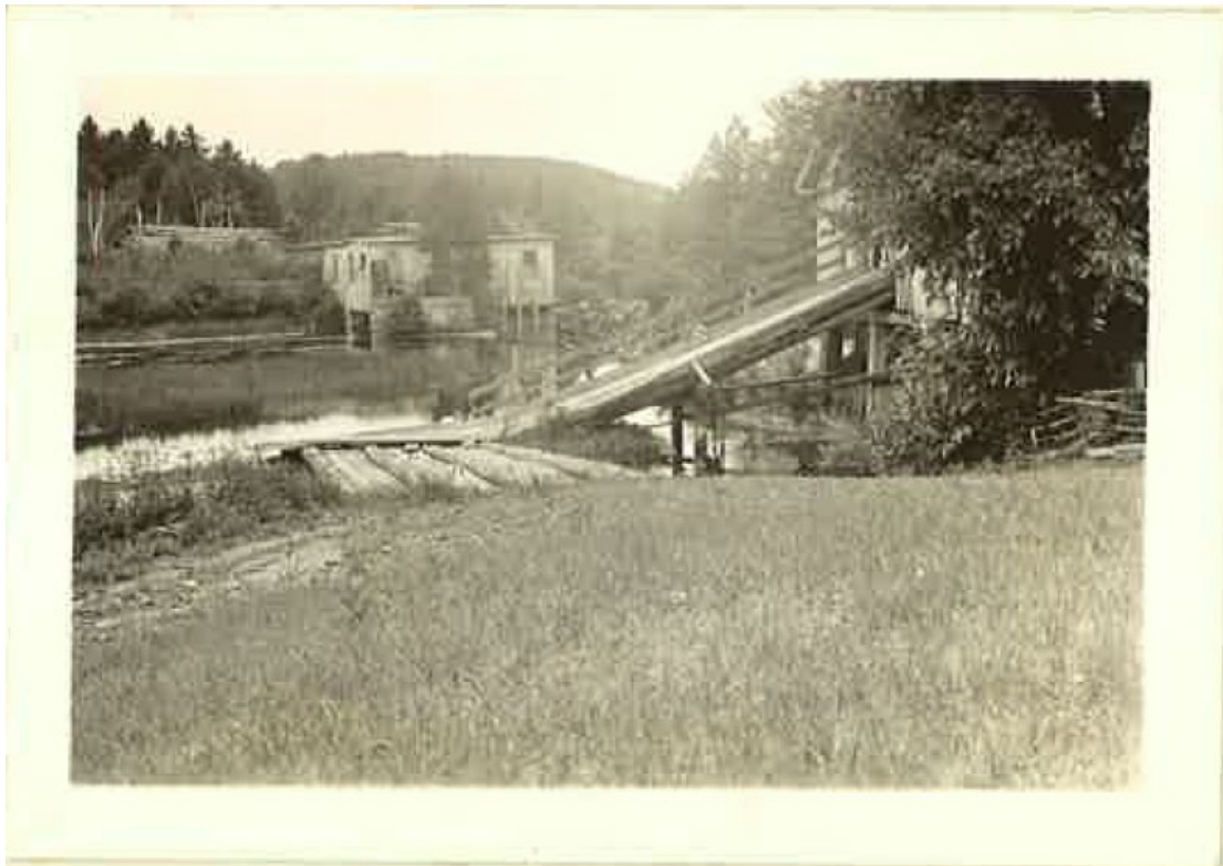
Figure 7. Rolfe Canal Dam (circa 1934 – removed in 1980)
