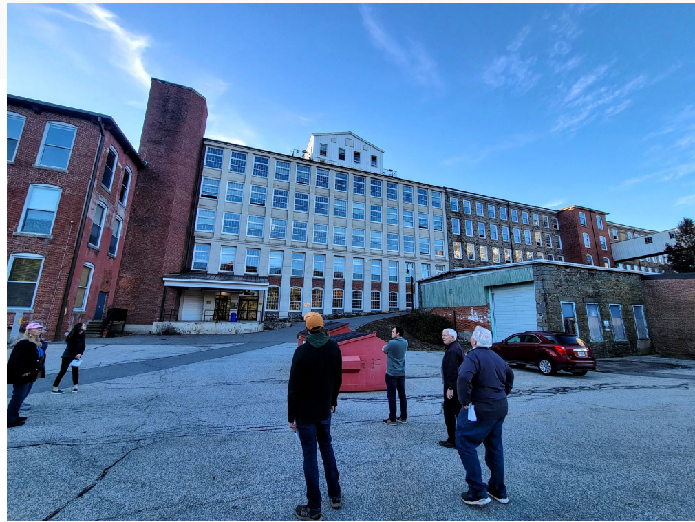
55 Main Street, Newmarket (The Millspace!)
