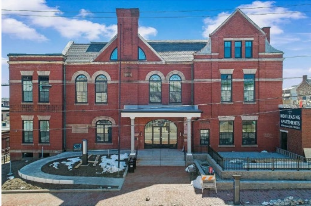
Former Strafford County Courthouse in Dover developed into housing.
