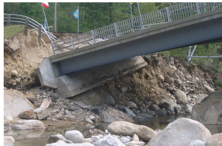
Loon Mountain Bridge Failure, Lincoln (Source: NH DES)
