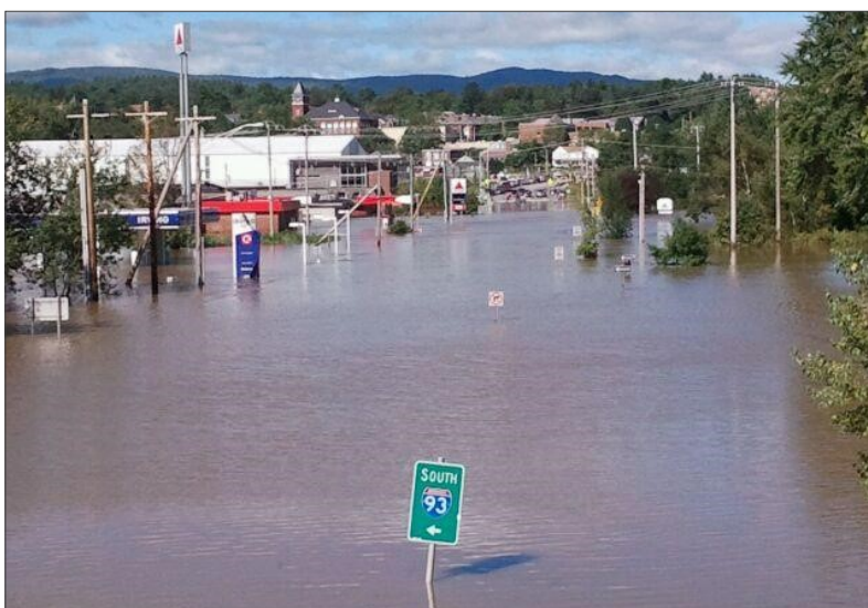
Flooding in Holderness Along Route 175 from Irene. (Source: Betsy Ayotte via Plymouth State )
