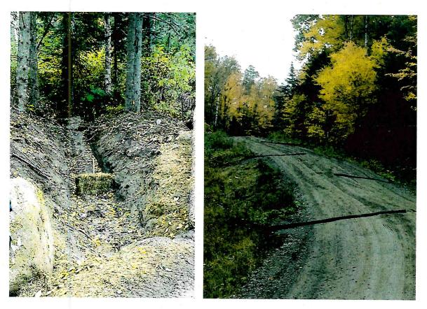
Figure 8 and 9- Picture on right shows the good exits of the newly installed culverts. Picture on left shows the rubber water diversion devices installed.
