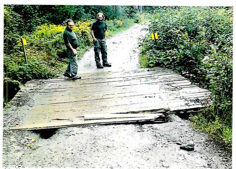
Figure 1, 2 and 3- Shows the broken boards on the bridges and the eroding approaches.
