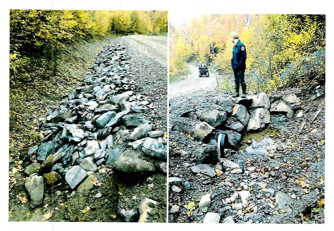
Figure 11 and 12- Depicts the newly fixed and armored ditch where the washout was previously. Also shows a newly installed culvert.
