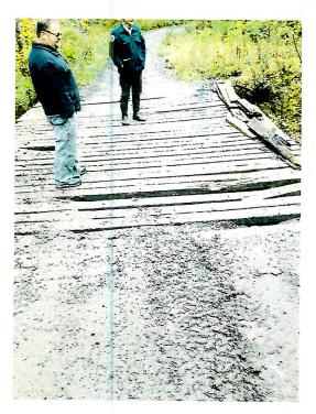
Figure 10- Depicts the repaired approach to the bridge, however, still shows the decking that needs replacing.
