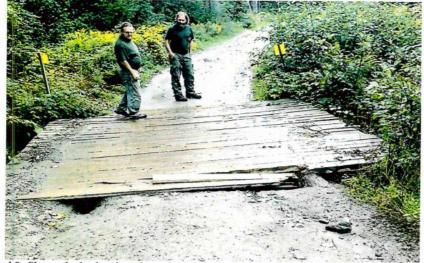
Figure 1, 2 and 3- Shows the broken boards on the bridges and the eroding approaches.
