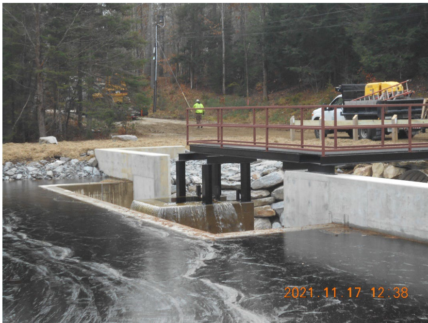
Photo 8: New Weeks Crossing dam looking southeast at road 11/2021.
