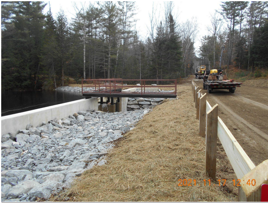
Photo 5: New Weeks Crossing dam looking southeast 11/2021.
