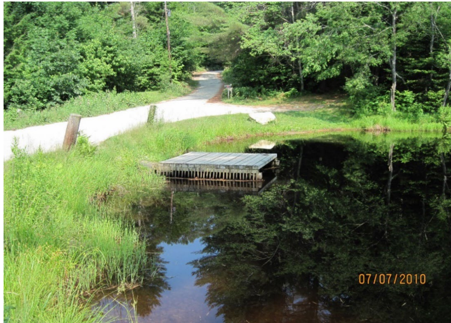
Photo 1: Weeks Crossing Dam looking northwest before failure. 7/2010
