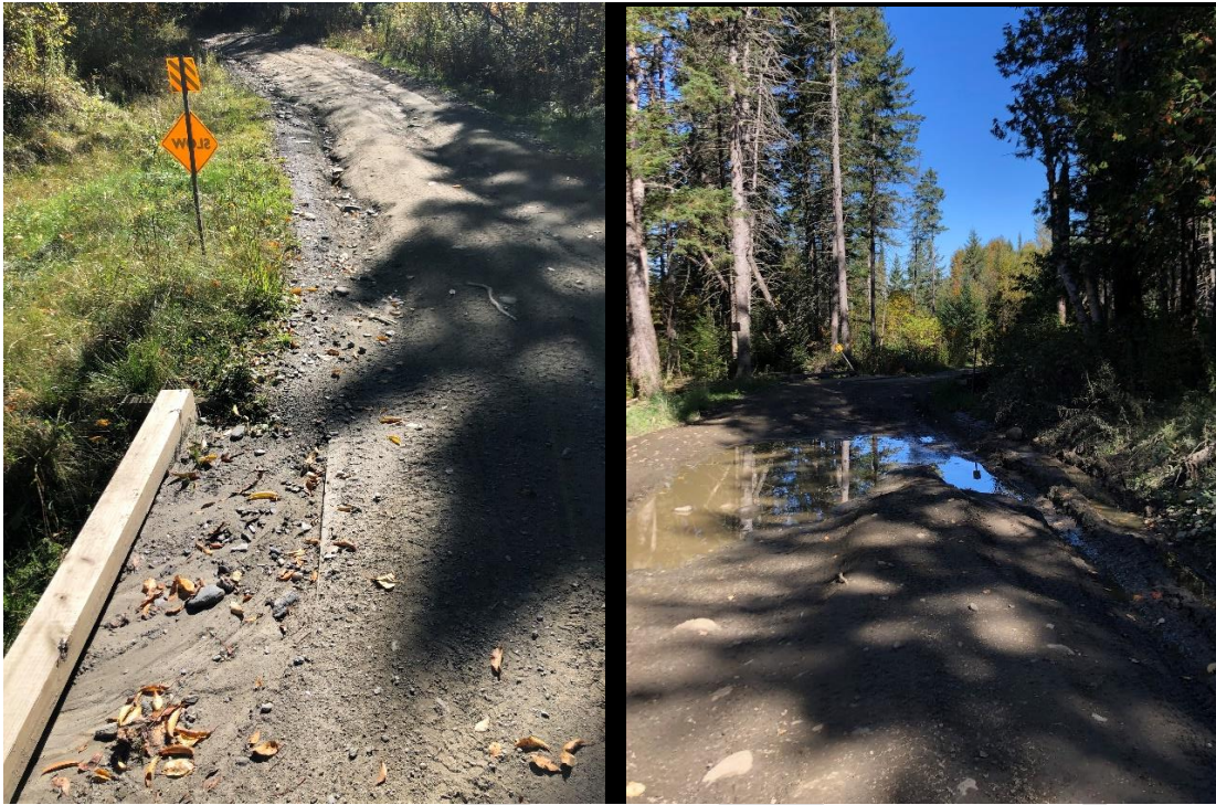
Figure 7- Shows sediment entering brook at bridge location and shows the “mud hole”
