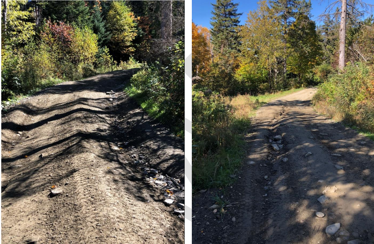
Figure 6- Shows condition of trail and some of the washing that had occurred.
