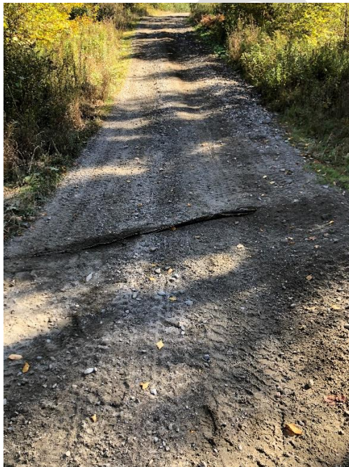
Figure 5- Shows the condition of the trail on the steep hill leading to the kiosk and the rubber water devices.
