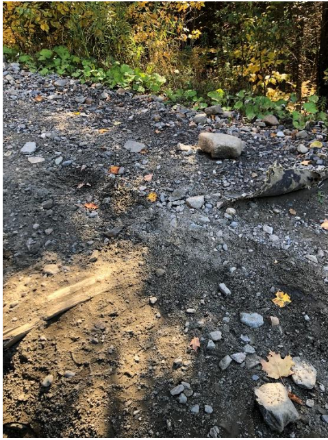
Figure 8- Depicting the rubber water diversion devices, where the rubber is completely missing.
