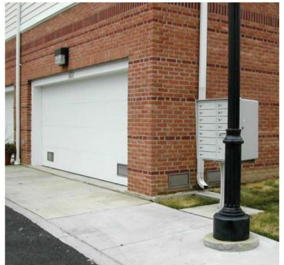
Figure 6: Engineered openings in garage doors
