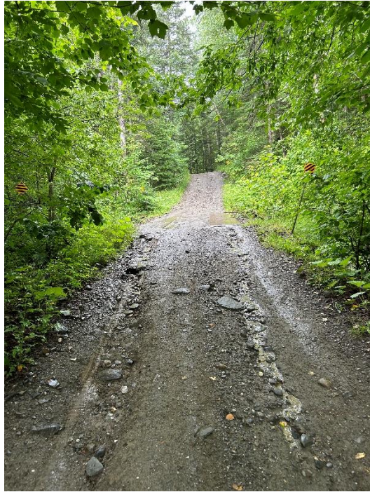
Figure 2 & 3- Depicts minor surface erosion after the July storm event
