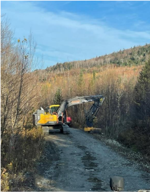
Figure 13 & 14- Illustrates the mowing along the trail with the Brontosaurus mulching head
