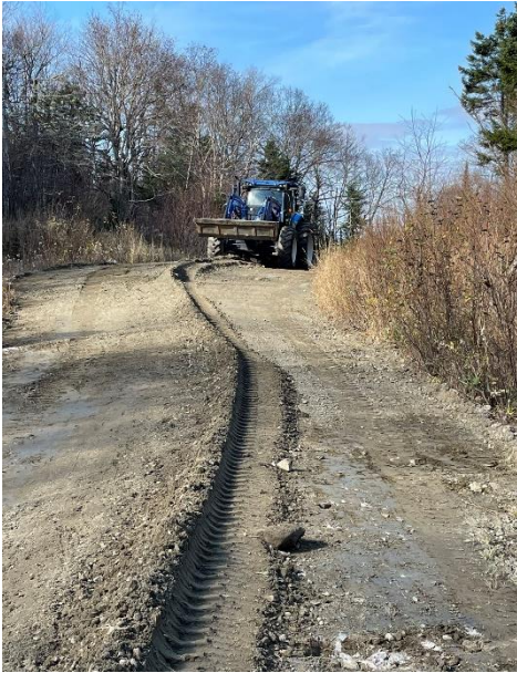
Figure 15 & 16- Depicts the rock crusher re-surfacing the road and existing conditions of trail.
