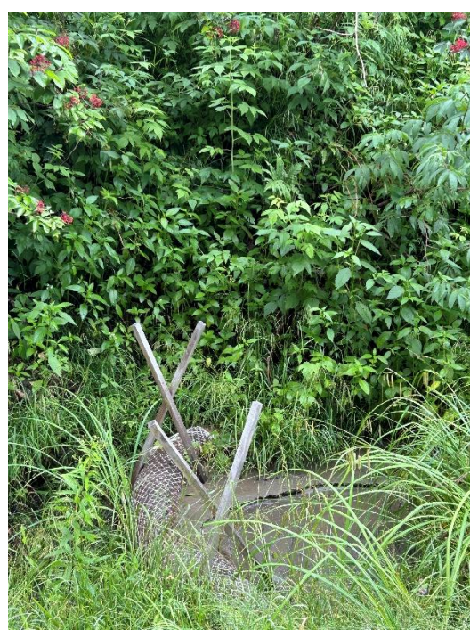
Figure 4 & 5- Depicts filled ditch lines and sediment traps from runoff
