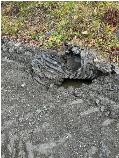
Figure 17- Depicts the culvert that was damaged during trail maintenance.
