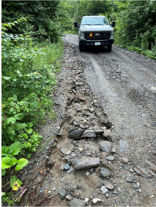
Figure 2 & 3- Depicts minor surface erosion after the July storm event
