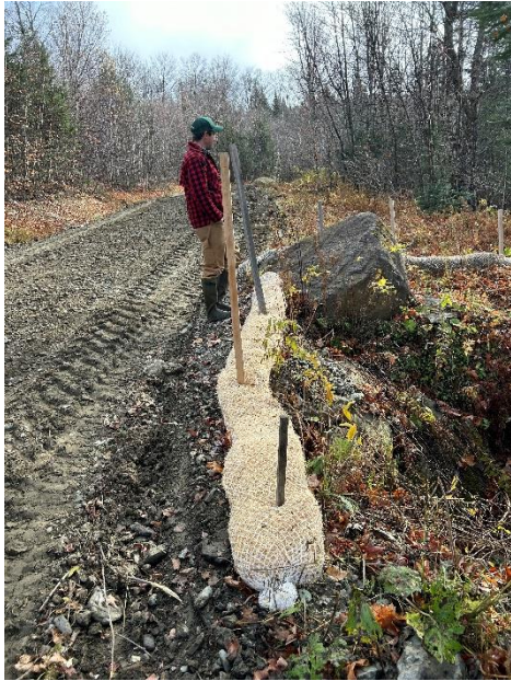
Figure 12- Depicts straw waddle added after the trail maintenance work to minimize erosion.
