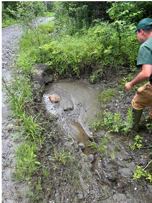
Figure 4 & 5- Depicts filled ditch lines and sediment traps from runoff
