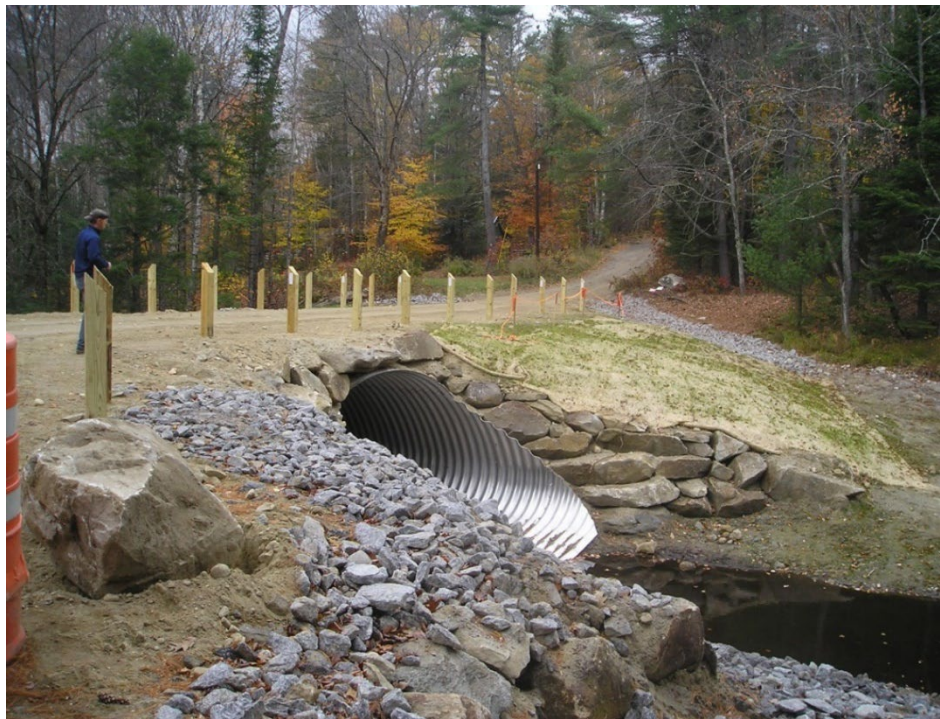
Photo 4: At repaired Gould Hill Road and culvert looking northwest 10/2018.
