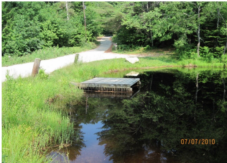
Photo 1: Weeks Crossing Dam looking northwest before failure. 7/2010
