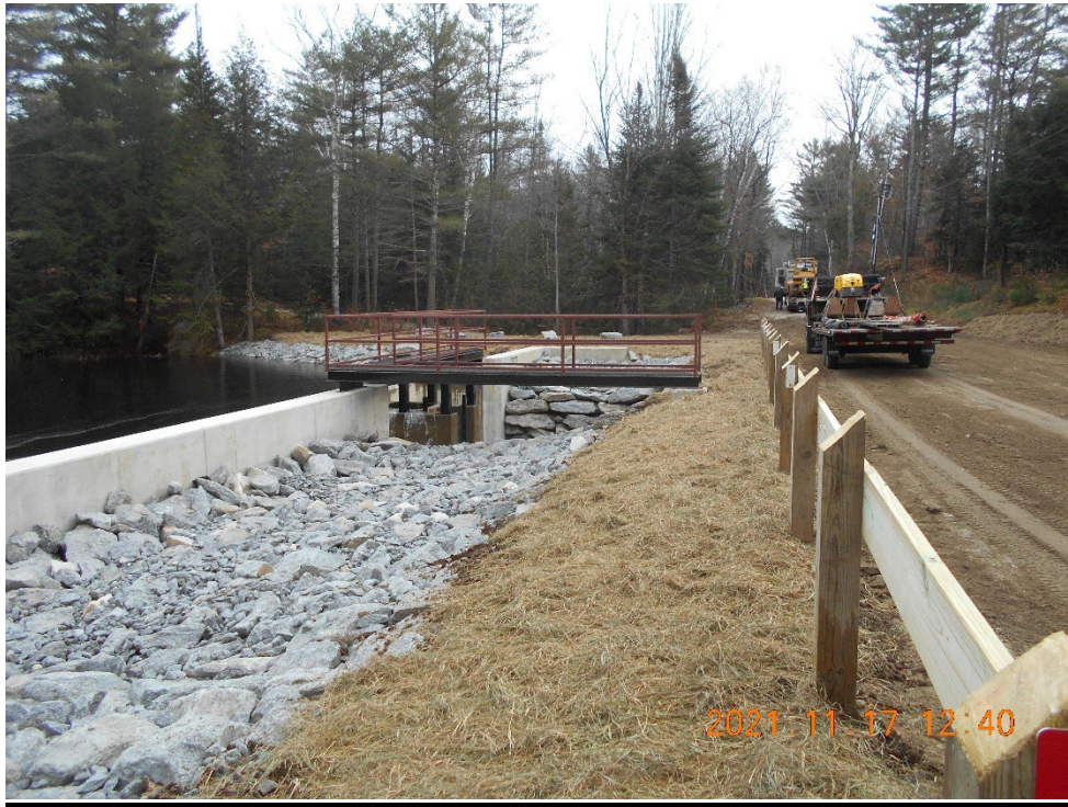
Photo 5: New Weeks Crossing dam looking southeast 11/2021.
