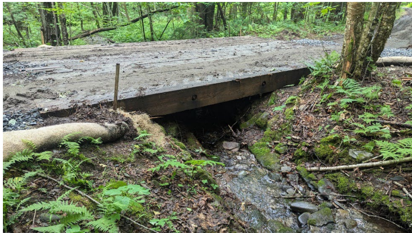
A new timber mat bridge at Lower Shaker WMA. Railings were installed later.
